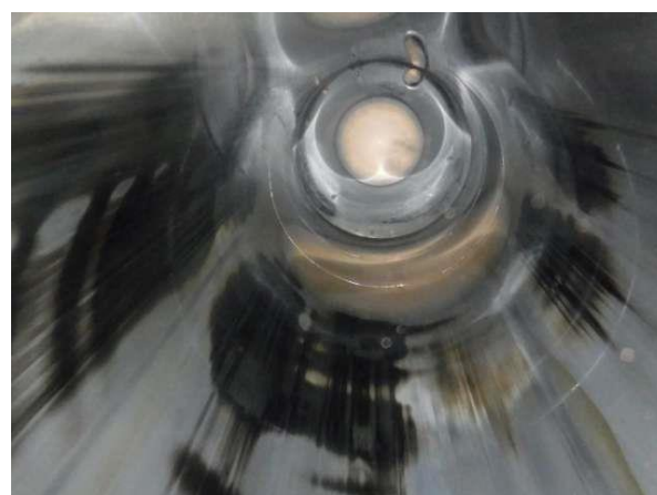
Signs of lacquering / black spots on cylinder liner walls
